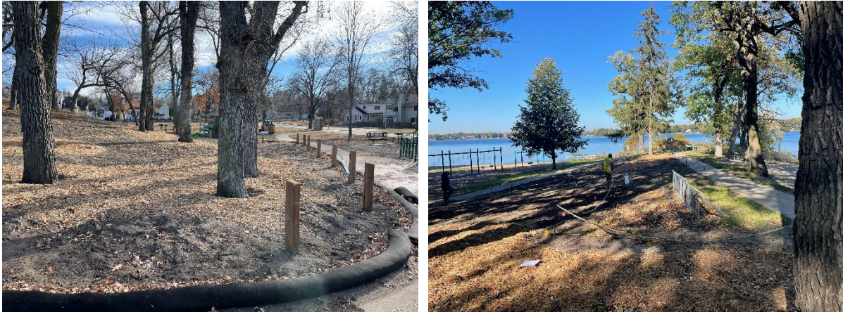
Photograph 10 & 11: Air spade, mulch, seeding and fencing being installed on the slope above the beach at The Commons, 2023
