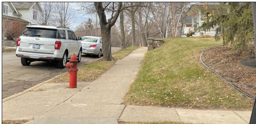
Photograph 12: Norway maple growing in Excelsior in a narrow boulevard, heaving the sidewalk adjacent near a fire hydrant
