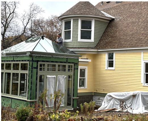
Recently approved addition to Landmark property with new design elements not historically present
